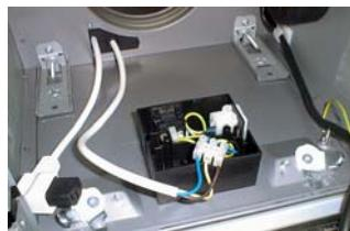
In presence of a yellow/green wire this has to be fixed to the earthing terminal of the hood. For what concerns the yellow/green wire of the remote blower it is necessary to fix it to the earthing terminal of the remote blower casing.
